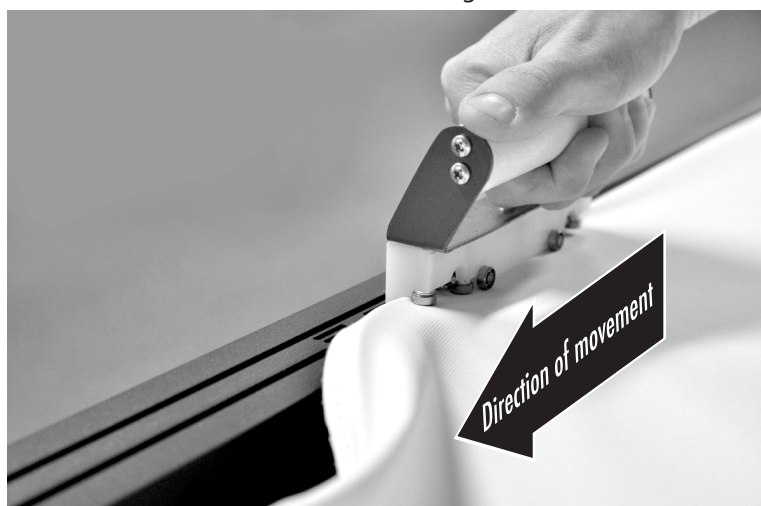
Front view of installing fabric with tool
