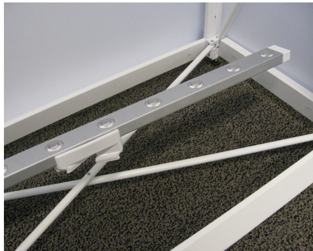
2. Align lightbar where frame bars cross each other.
