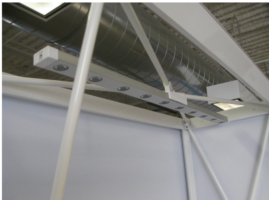
2. Align lightbar where frame bars cross each other.
